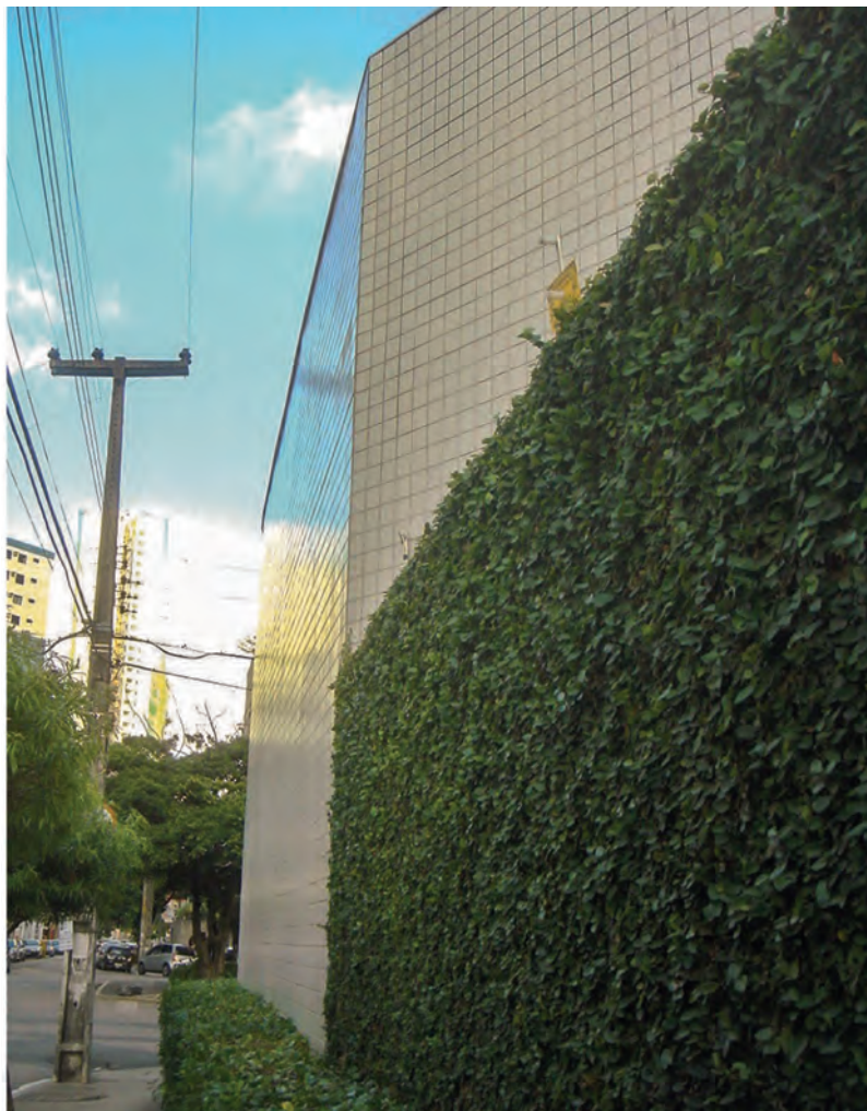
Large car park walls of buildings constructed in the 1990s. Setback with vegetation required by 12 Neighborhoods Act. Building characteristic of the 1980s. PHOTOS: collection of Geraldo Marinho
