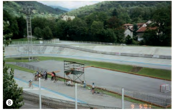
FIGURE 1 Detention basins used for sports and leisure on days without rainfall. A) Porto Alegre (Brazil), B) Grenoble (France).
