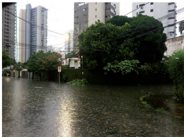
FIGURES 5 AND 6 Hillsides exposed to landslides in Nova Descoberta, Recife, 2021, and flooded streets in Casa Forte, Recife, 2020. Examples of disasters involving water.
